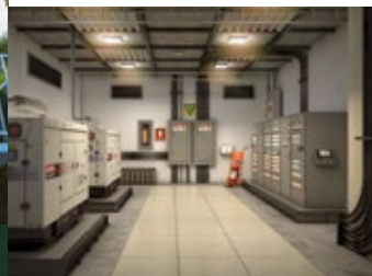
Provision of 100% Power back-up 24*7
