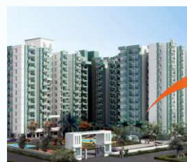
HIGHEND PARADISE 260 BHK Apartments at Rajnagar Extn., Ghaziabad Delivered
